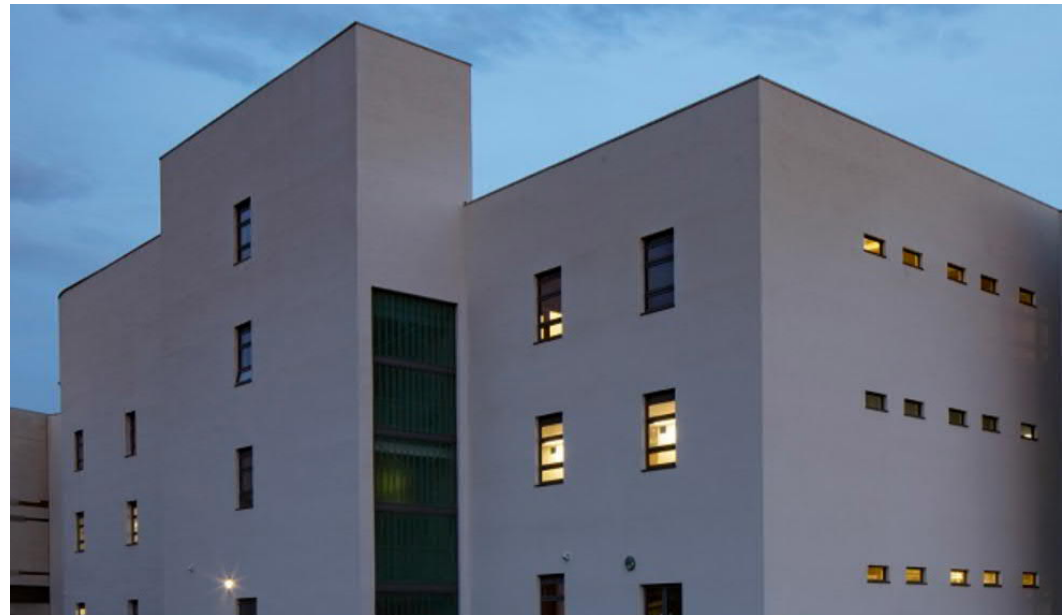
Northumbria Specialist Emergency Care Hospital
